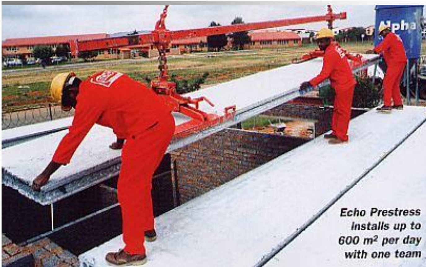
Pre-cast pre-stressed hollow core slab section (SA Builder Bouer, 2004b)
