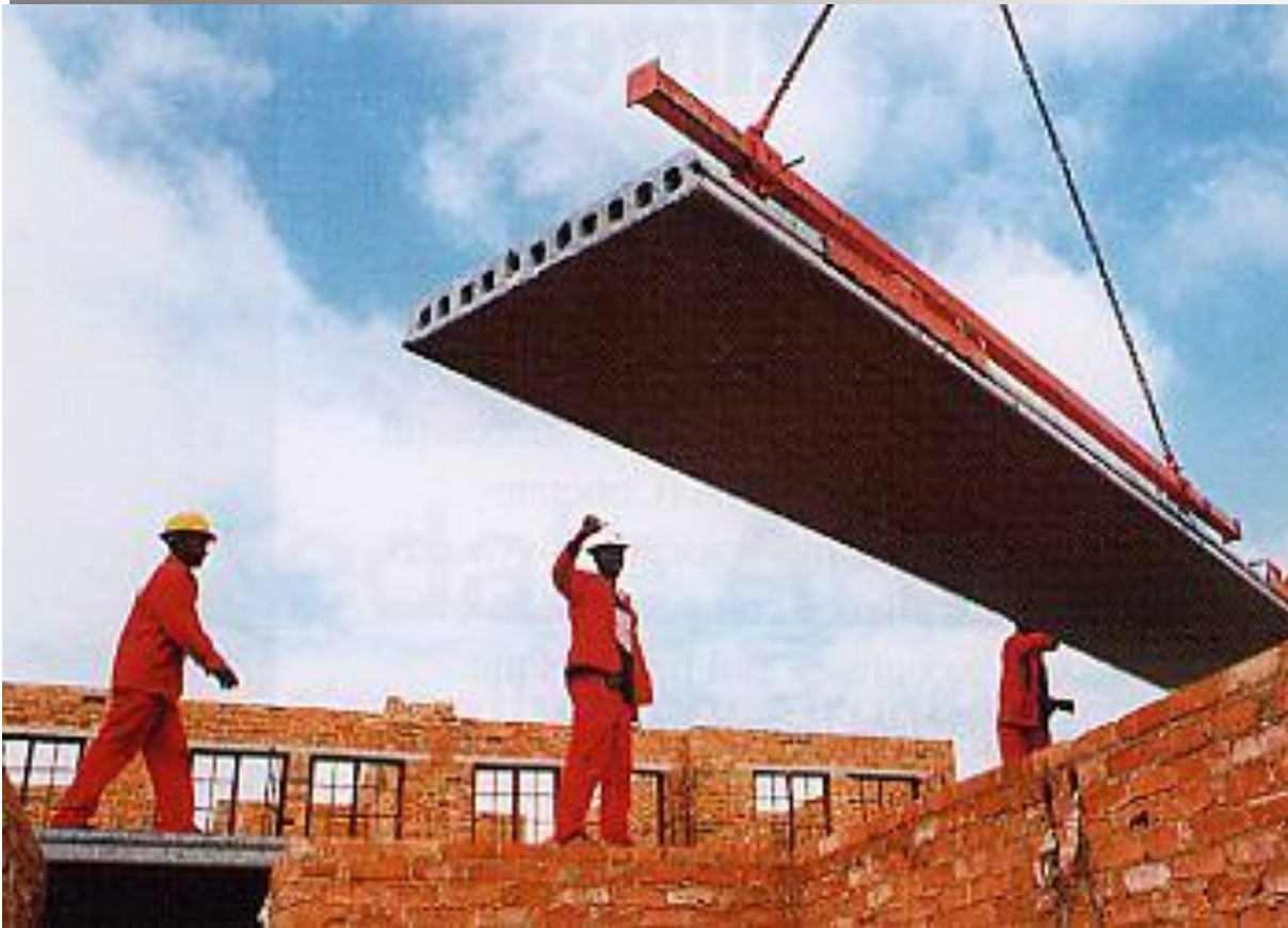
Pre-cast pre-stressed hollow core slab section (SA Builder Bouer, 2004a)
