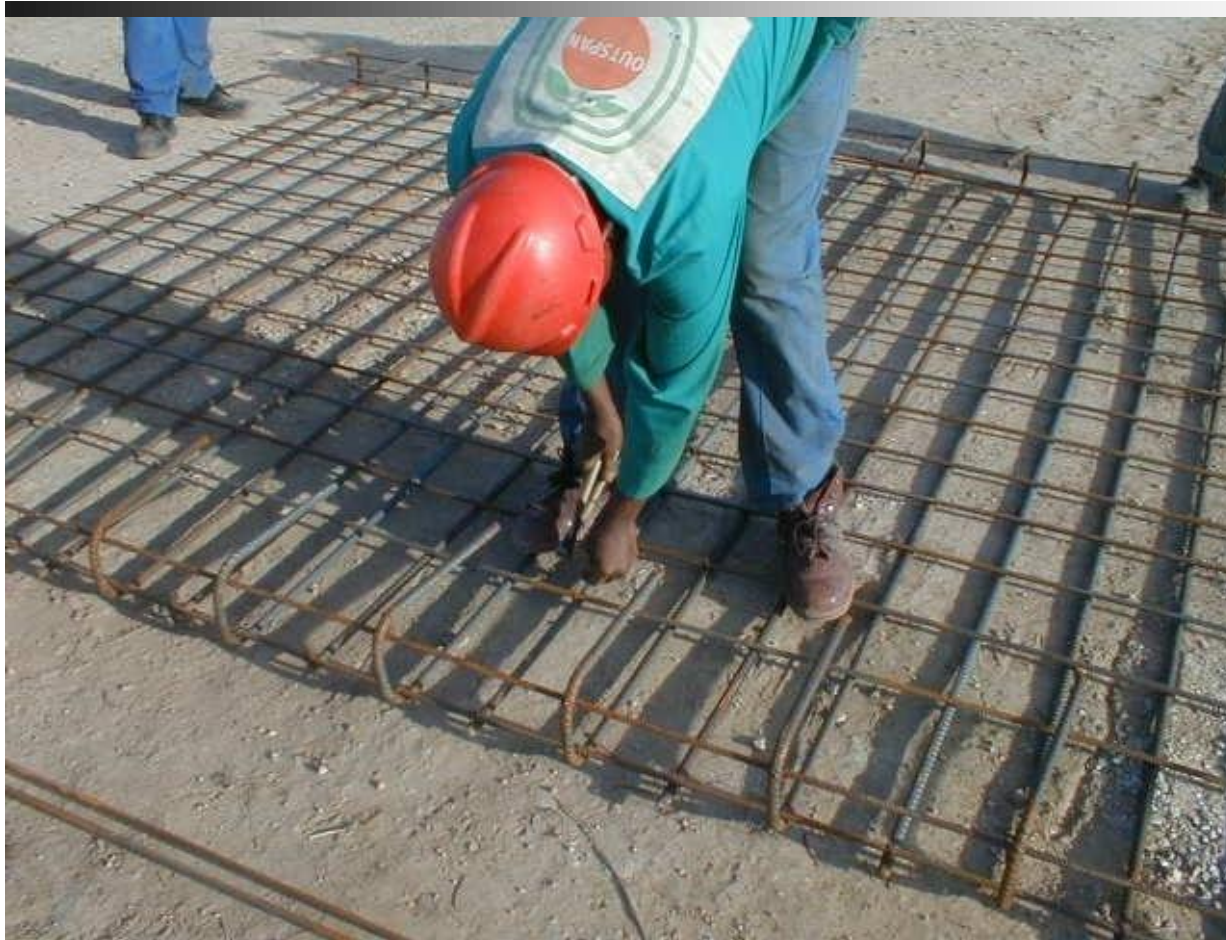
Tying reinforcing – bending, rapid repetitive movements etc. (Deacon, 2004)
