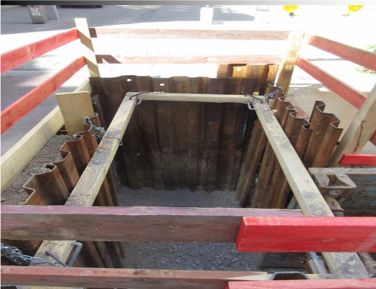
Shoring, Munich, Germany (Smallwood, July 2019)
