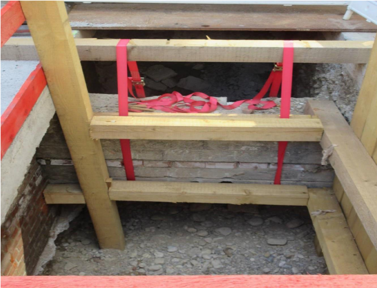
Shoring, Munich, Germany (Smallwood, July 2019)
