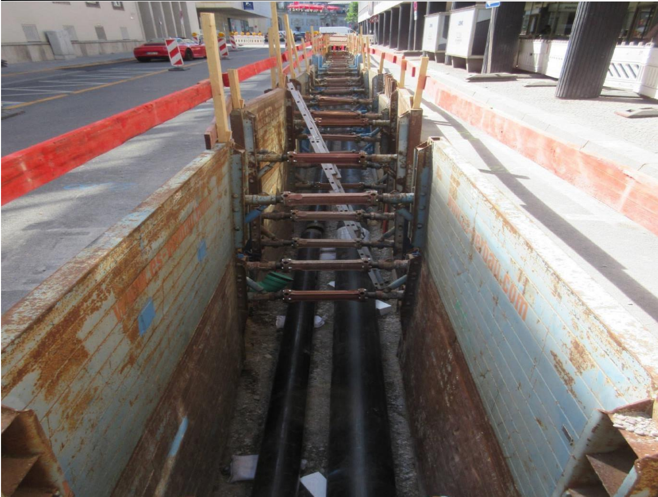
Shoring, Munich, Germany (Smallwood, July 2019)
