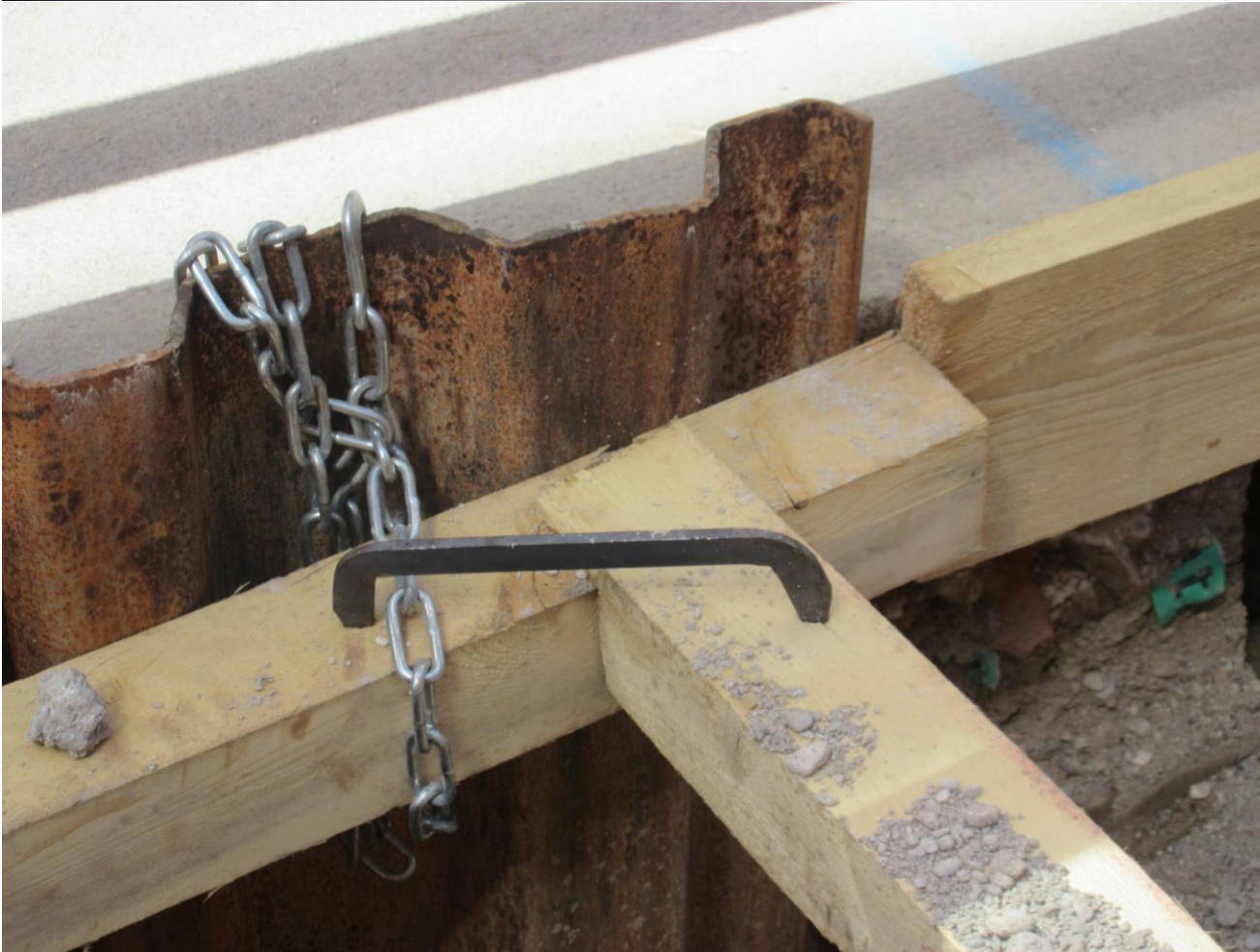
Shoring, Munich, Germany (Smallwood, July 2019)
