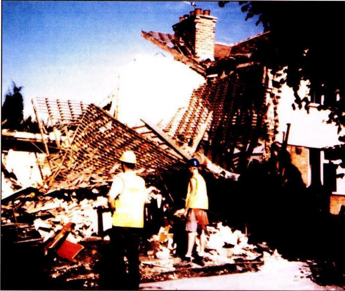
Aftermath of a gas explosion following damage to an underground gas service pipe (HSE, 2000)
