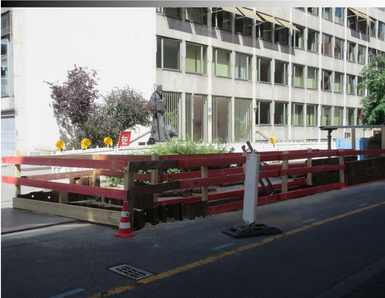
Barricading to excavations, Munich, Germany (Smallwood, July 2019)
