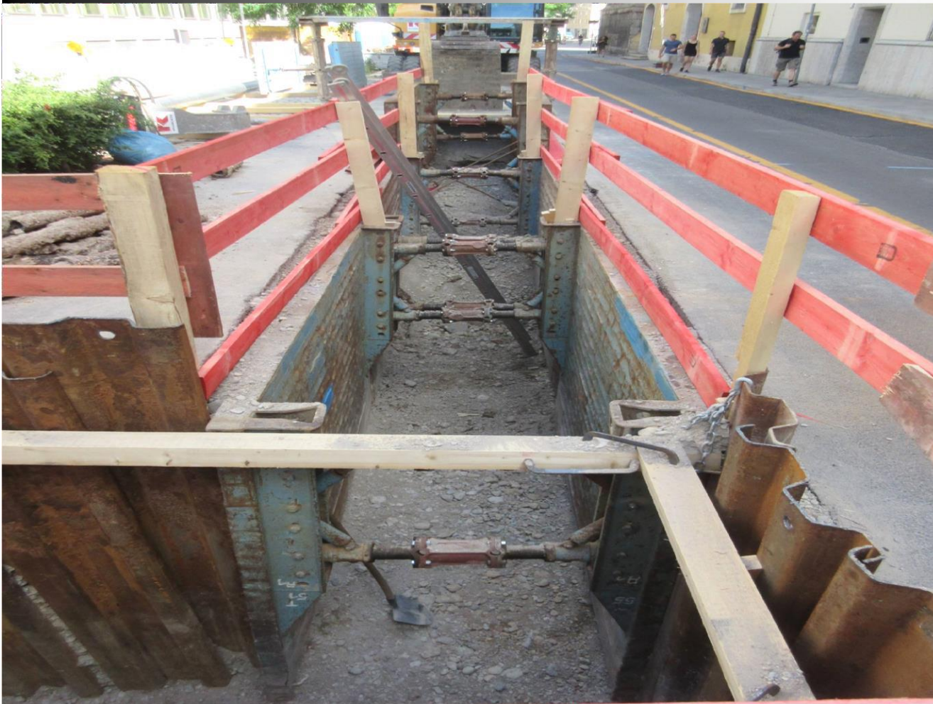
Shoring, Munich, Germany (Smallwood, July 2019)
