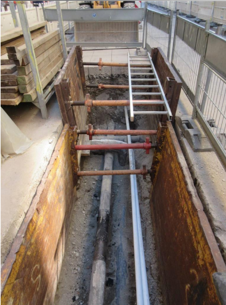
Shoring, Munich, Germany (Smallwood, July 2019)
