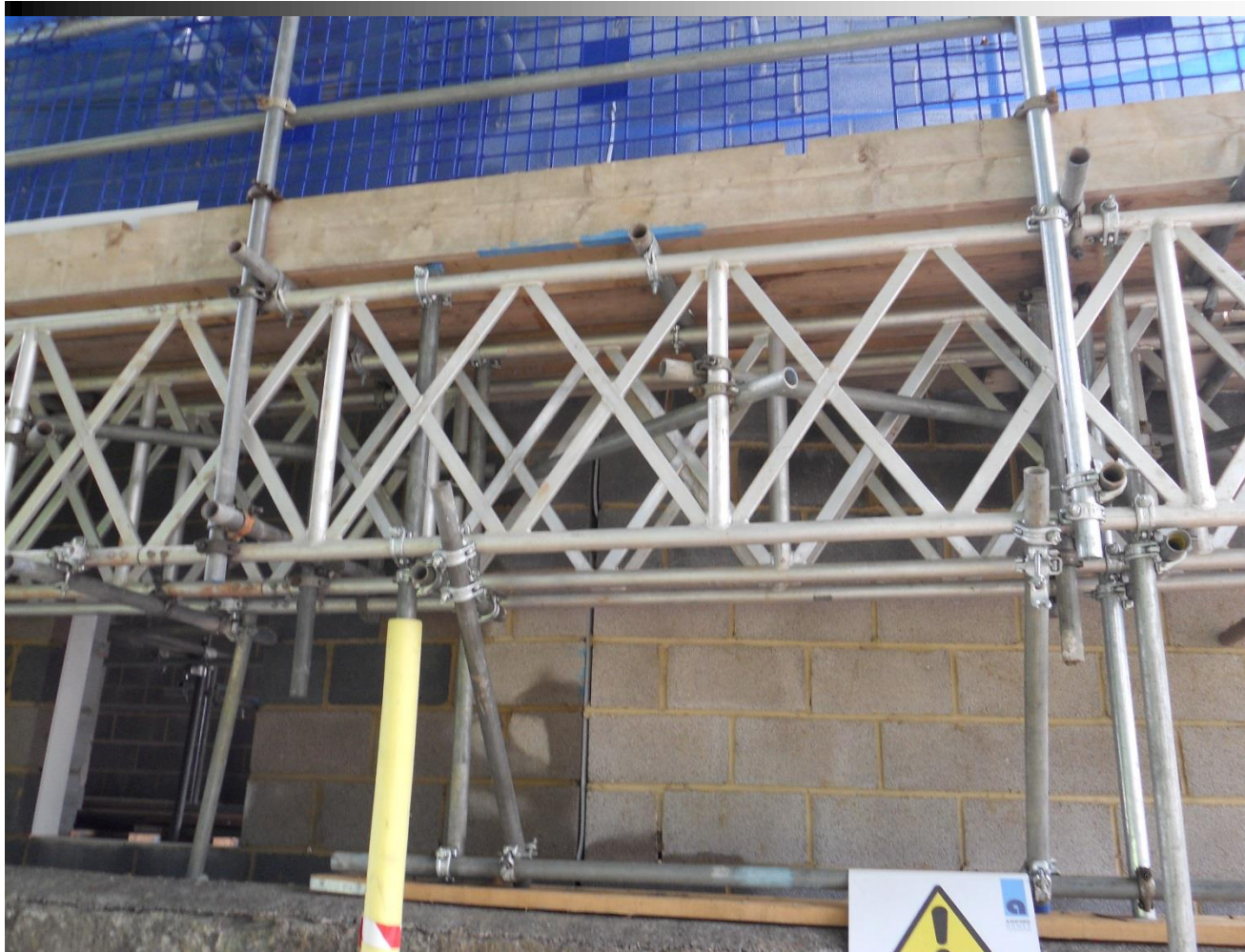
Scaffolding, Bradford on Avon (Smallwood, August 2014)
