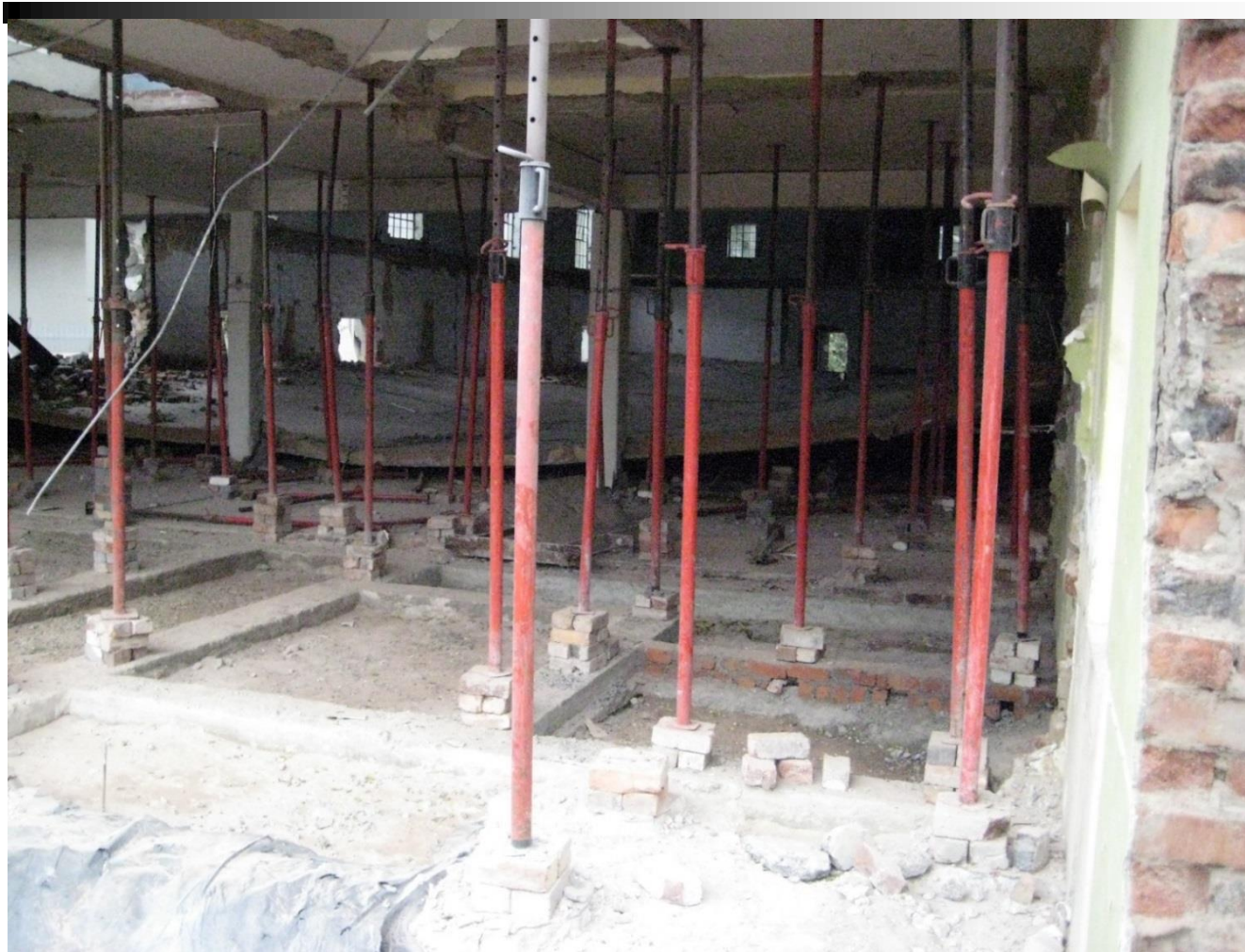
Stellenbosch Collapse (Anonymous, June 2008)
