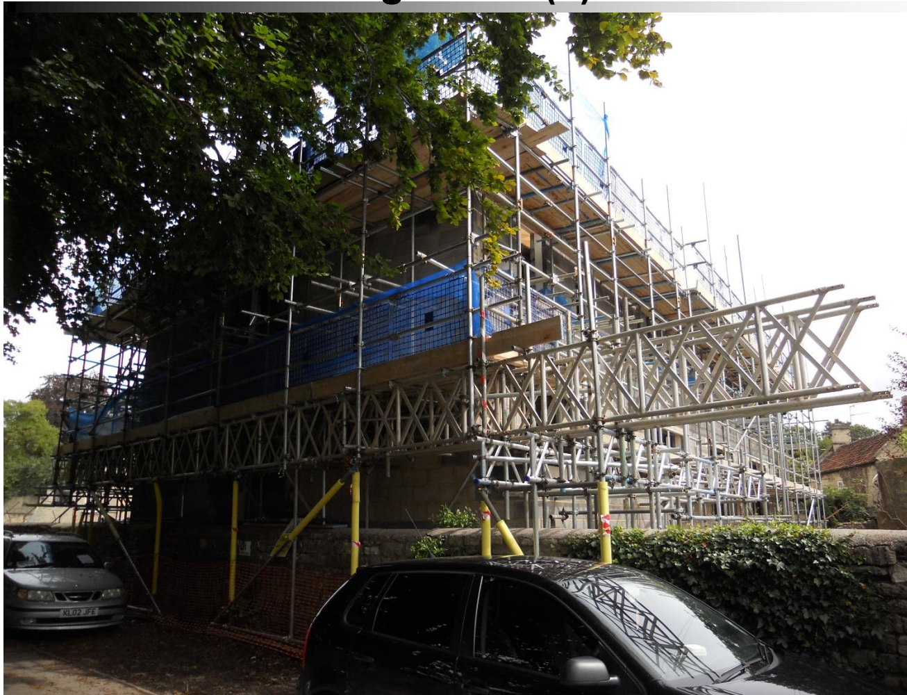
Scaffolding, Bradford on Avon (Smallwood, August 2014)
