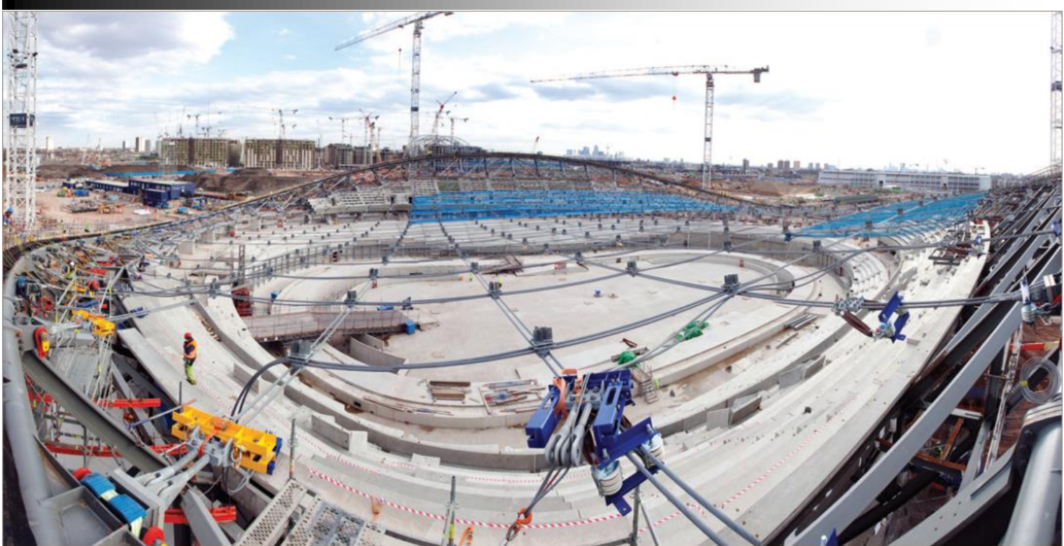
Alternative cable-net roof for the Velodrome (Shiplee, Waterman, Furniss, Seal and Jones, 2011)
