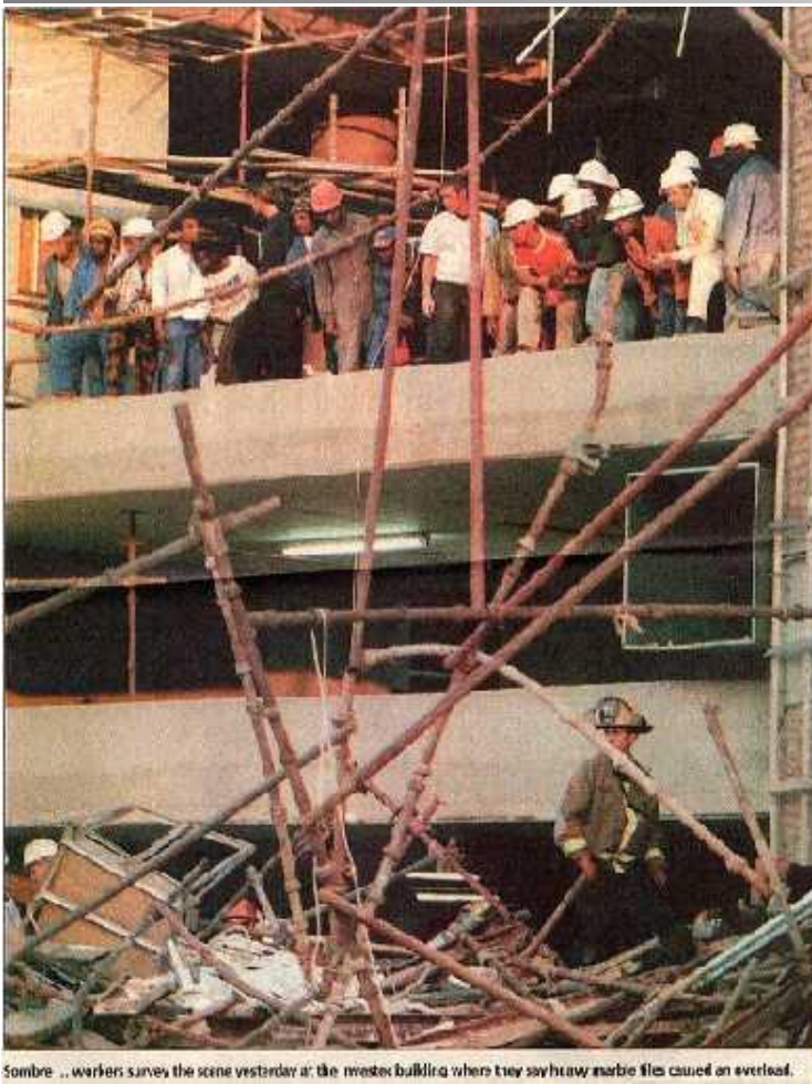
Investec Office Complex scaffolding collapse, Sandton, August, 1997 (Nesbitt, 1997)
