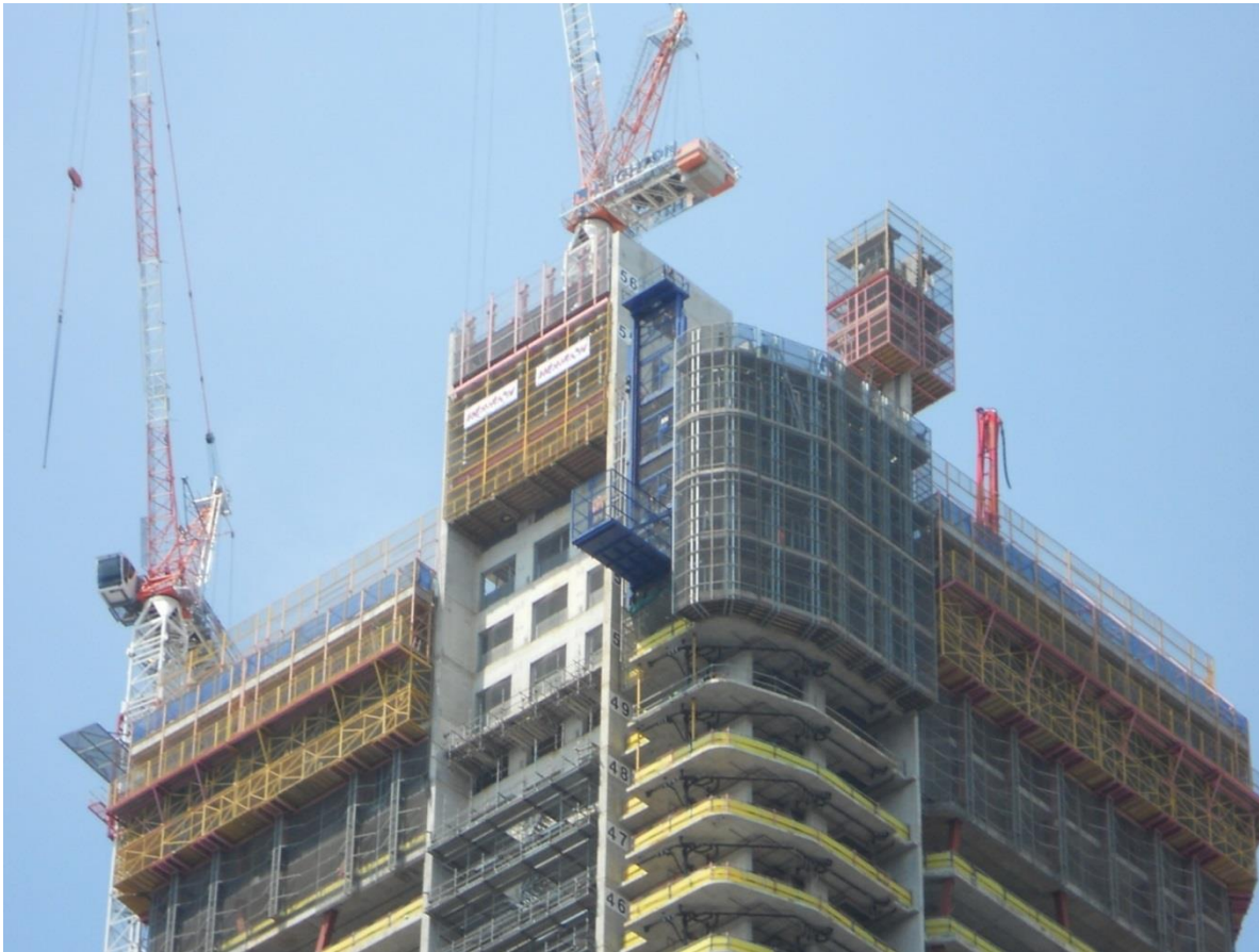
Tower cranes, Brisbane, Australia (Smallwood, 2011)
