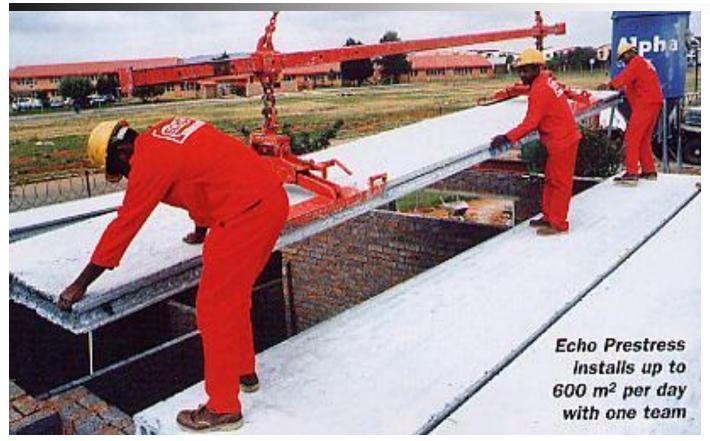
Pre-cast pre-stressed hollow core slab section (SA Builder Bouer, 2004b)
