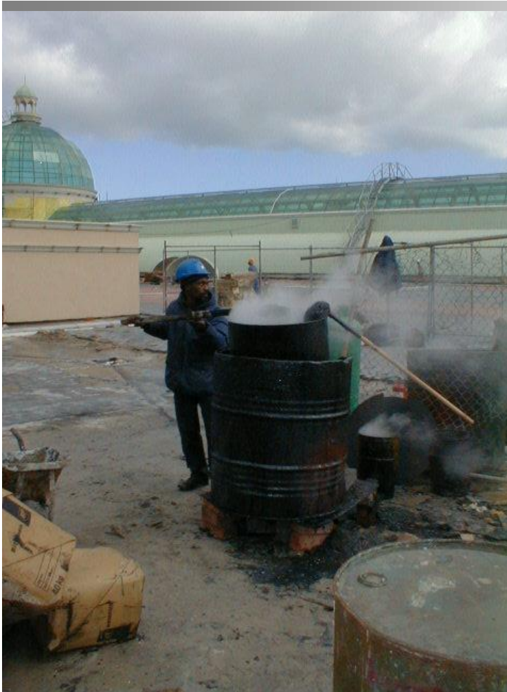
‘Melting’ mastic asphalt (still available), Canal Walk, Cape Town (Smallwood, 2000)
